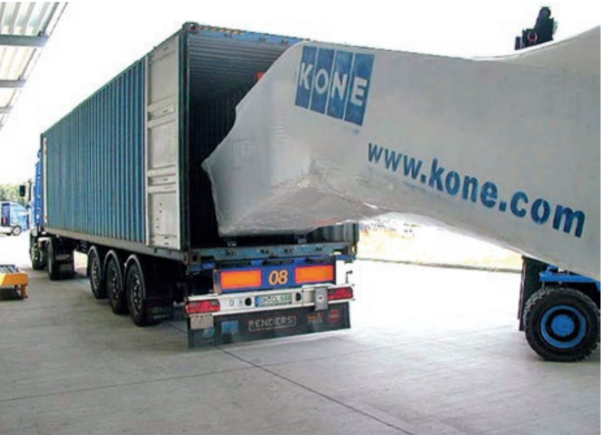
Figure 7.7 Unloading an escalator using forklift trucks
