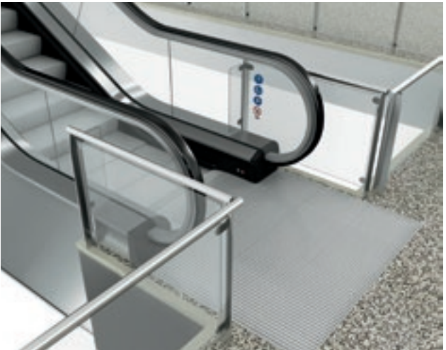
Figure 5.17 Standard arrangement without extended balustrade requires 90° static railings to be installed for safety reasons
